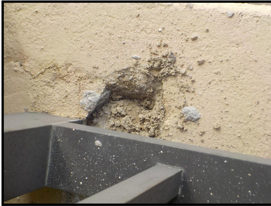
Example of original pocket-fill material.
