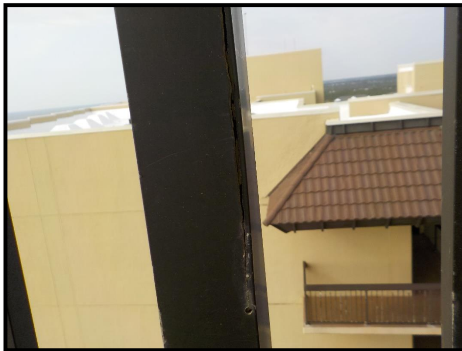
Cracked/split metal stanchions (likely from freeze/thaw cycles) on the West side of the balcony area.
