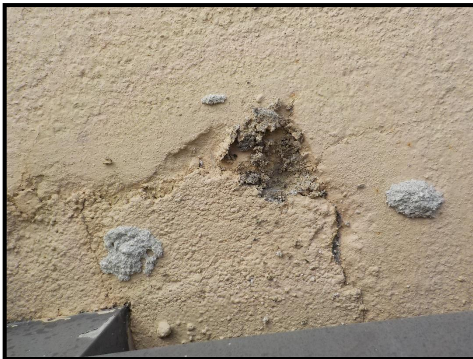
Example of difference in material between original pocket-fill and “cap” repair material.
