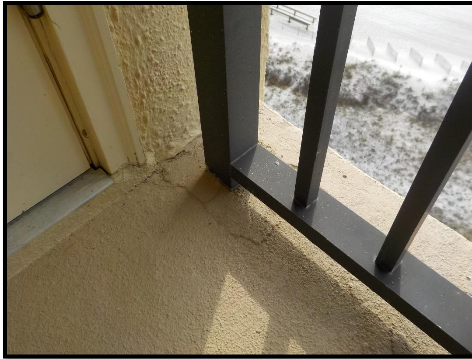
Stanchion with stanchion pocket “cap” repair rather than a full in-depth repair.
