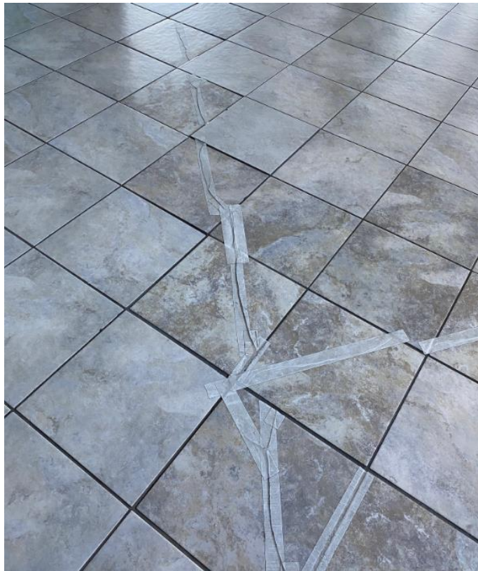
Figure 2: Front Lobby Tile Cracking
