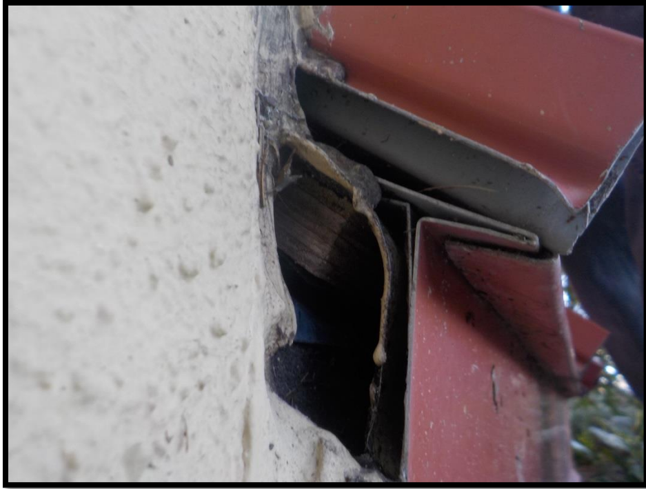
8 – Close up of exposed lumber beneath roof.
