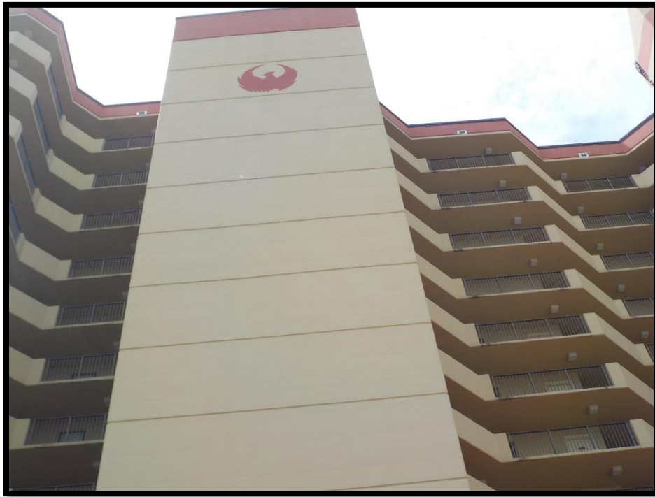
1 – Overview of building face. Lack of sheen and faded coloring.
