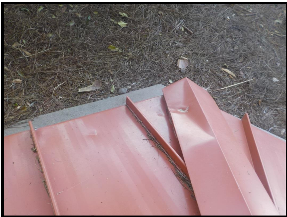
8 – Impact damaged ridge cap.
