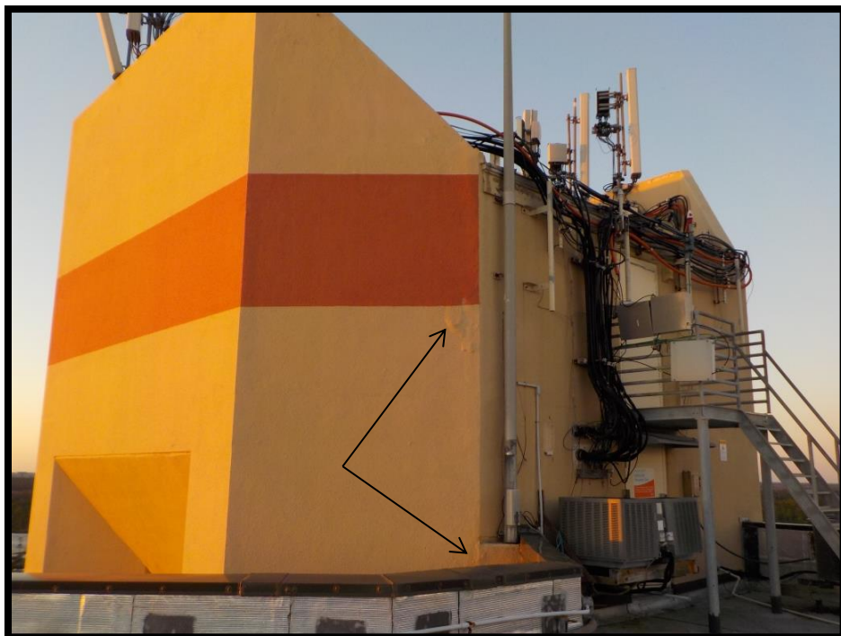
Elevator penthouse. Note coating blisters.
