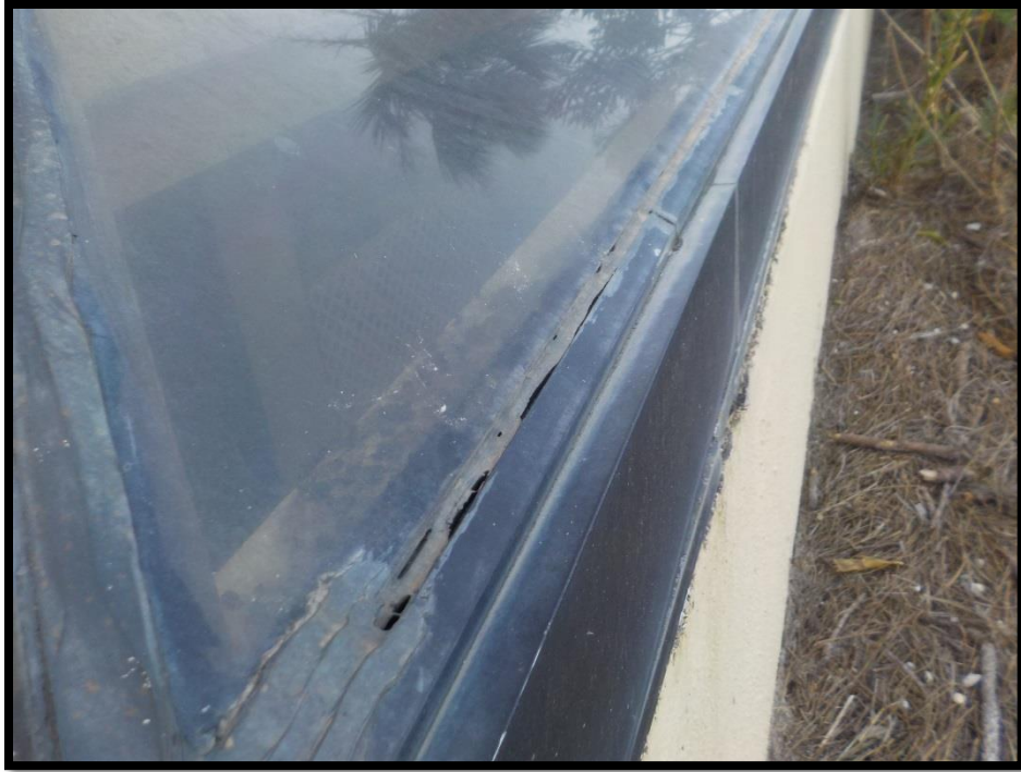
8 – Sealant failure at skylight.
