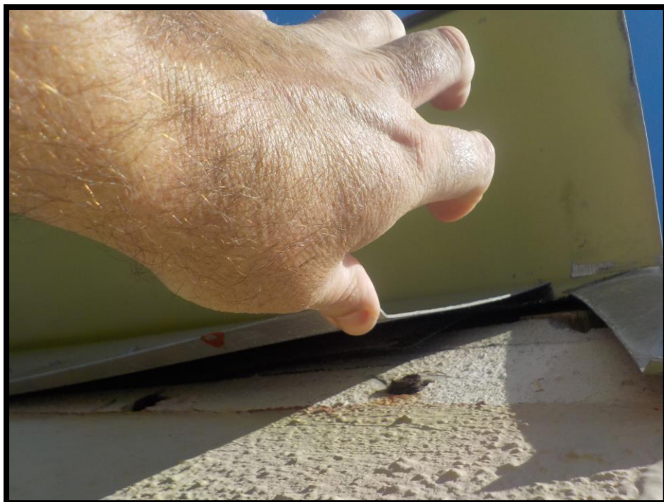
Exposed penetrations just behind stairwell penthouse flashing.
