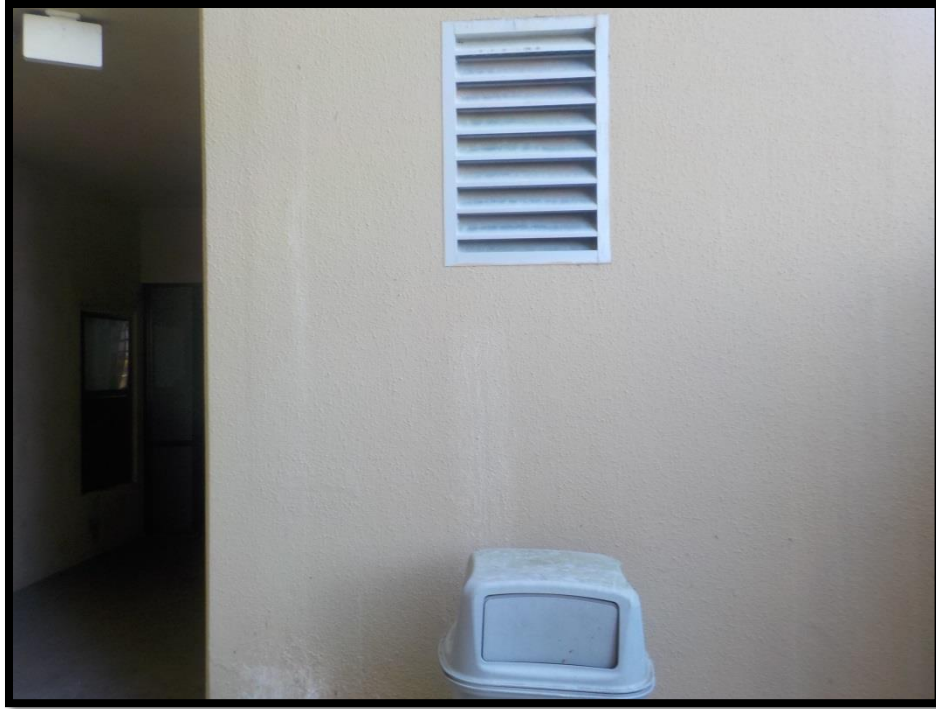
2 – Efflorescence on wall coating below vent.
