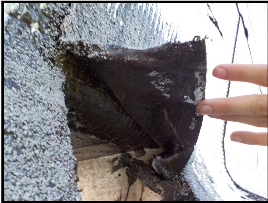
Scupper throat flashing condition observed.
