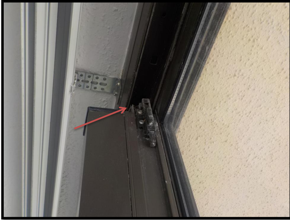
36 - Note door position in reference to interior frame when pushed toward exterior.
