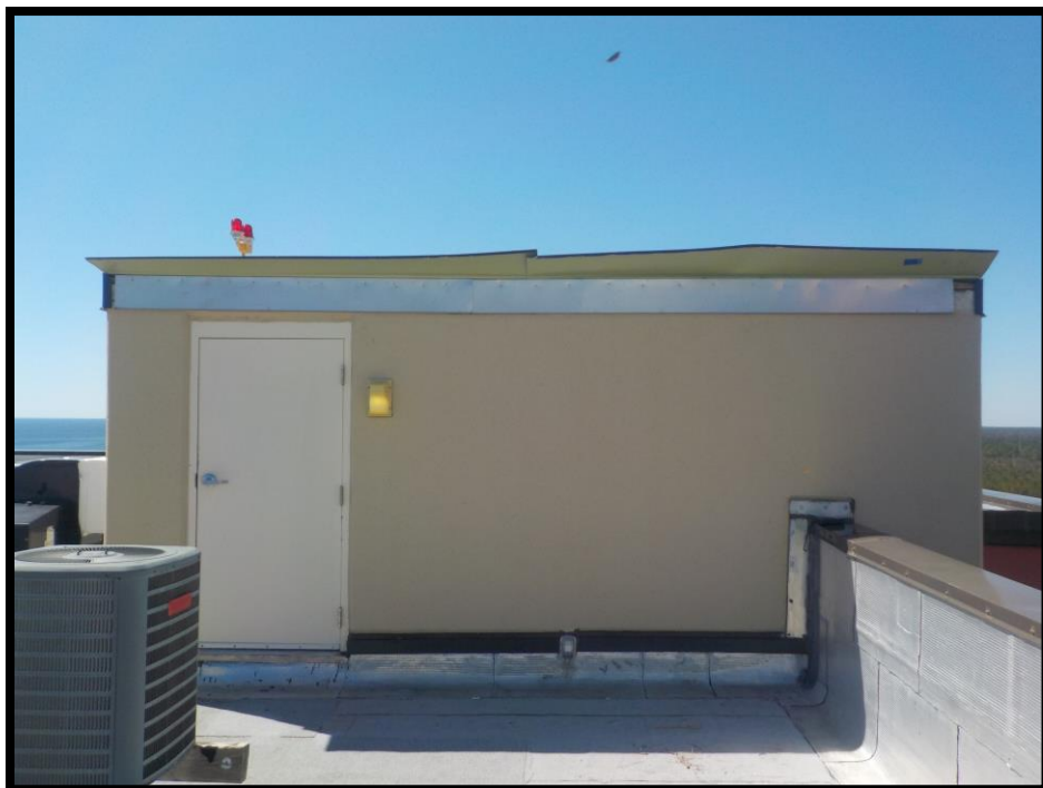
Stairwell penthouse flashing damage.
