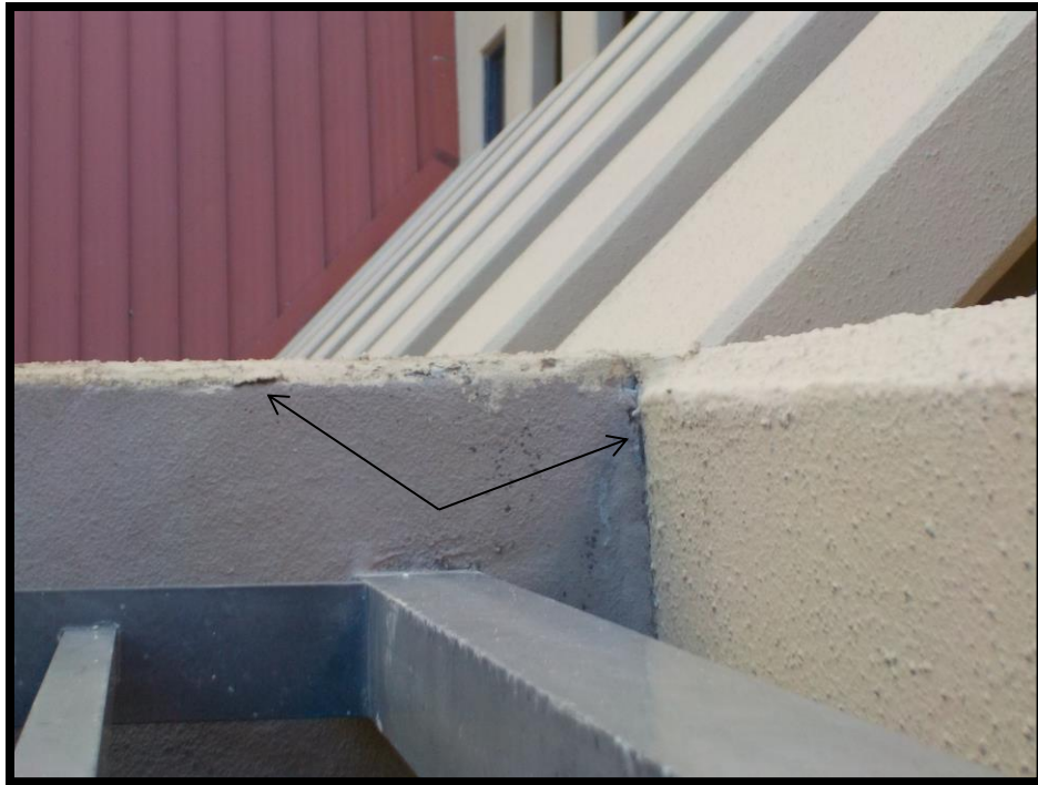
25 – Openings at coating abutments with wrinkling of slab face coating.
