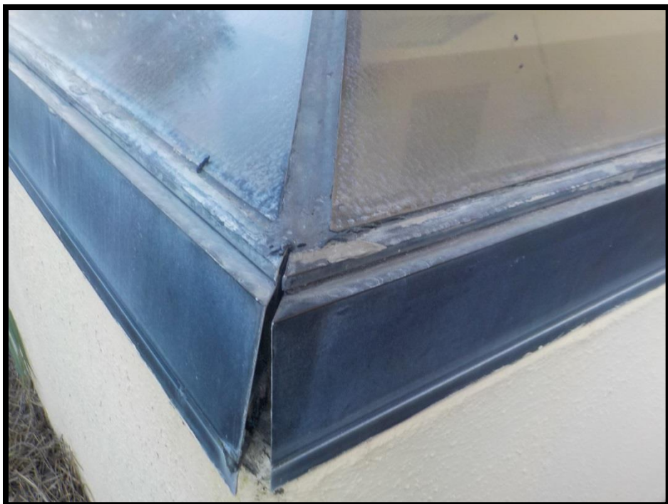
1 – Skylight framing separation.
