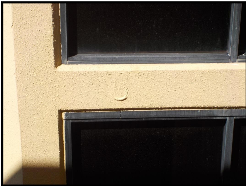
7 – Vertical wall blister beneath an elevator penthouse window.
