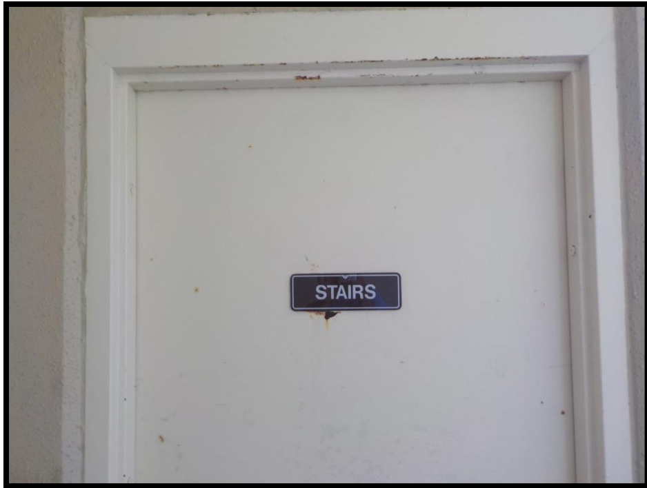
5 – Door and frame in early stage of corrosion.
