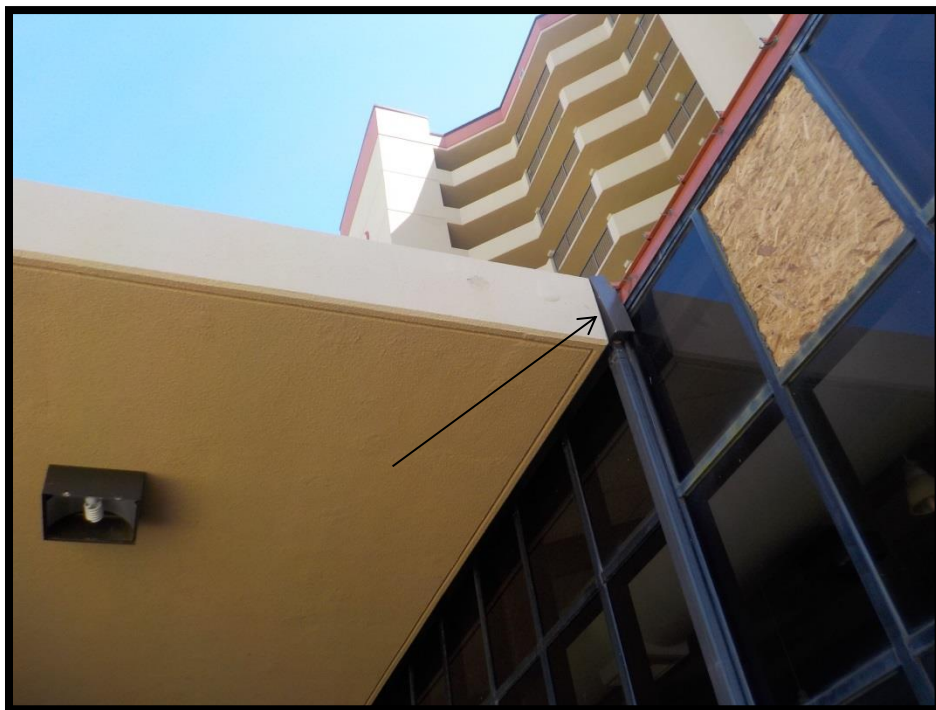
3 – Hurricane damaged window. Also note loose metal at window frame to roof.
