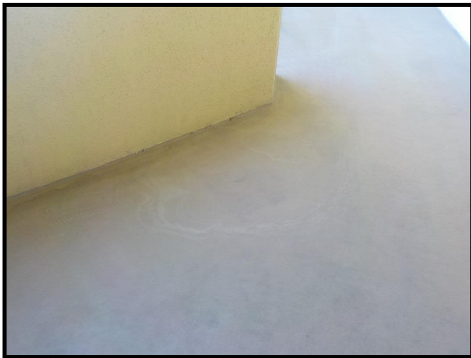
2 – Deck puddle evidence. Typical against common walkway knee walls.
