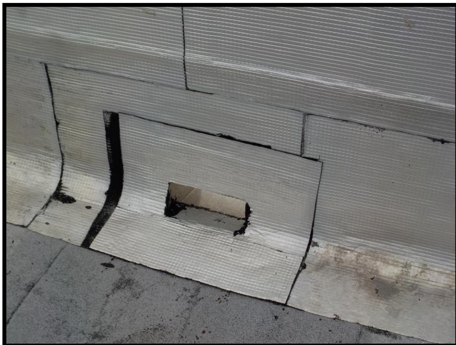
Example of roof overflow scupper.
