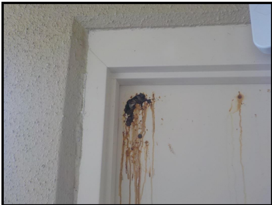
5 – Door skin corroded through.
