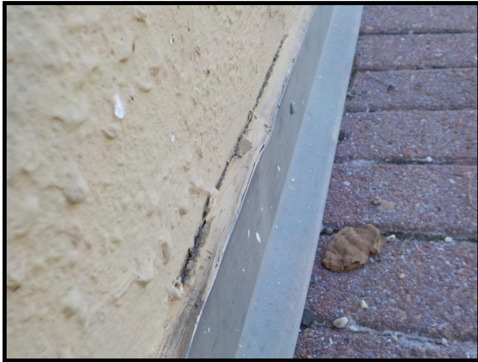
5 – Failed flashing sealant.
