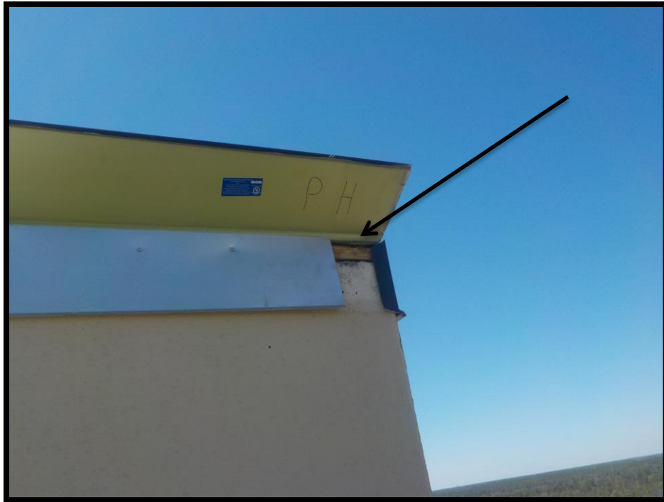
Note exposed lumber and lack of flashing lap.
