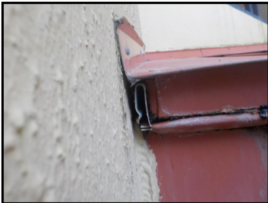
8 – Close up of open roof to wall termination.
