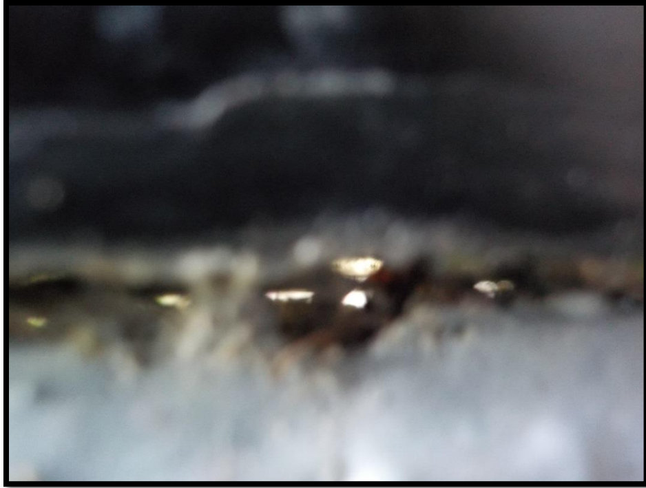
3 – Daylight from interior to exterior at curtain wall perimeter.
