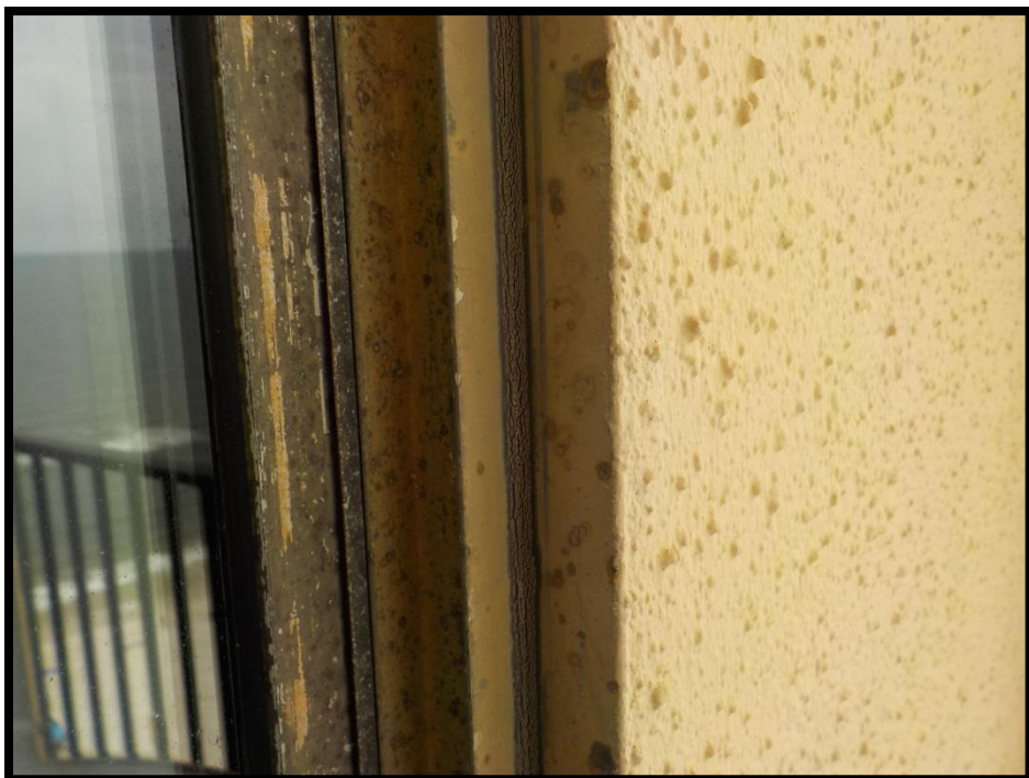
8 – Sealant failure at a South window.
