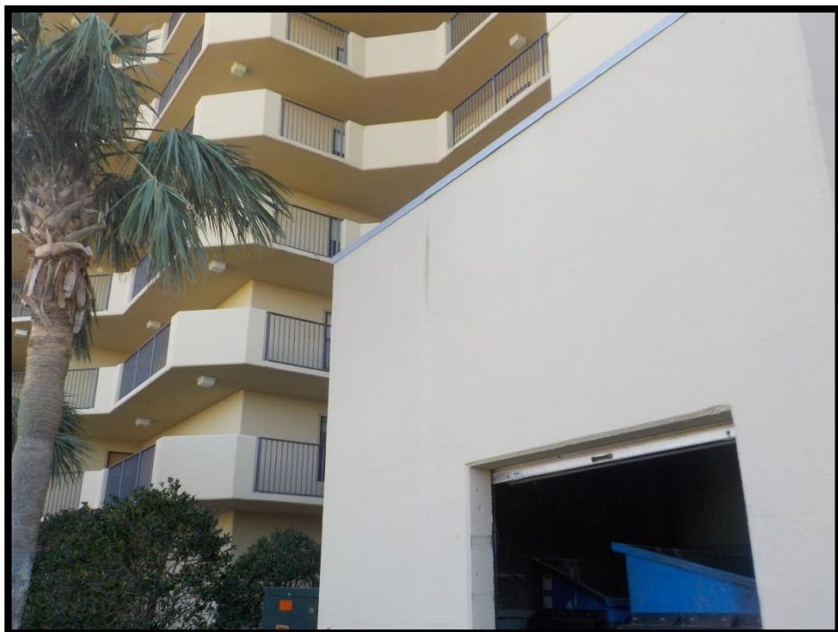
4 – Moisture stain below coping cap joint.
