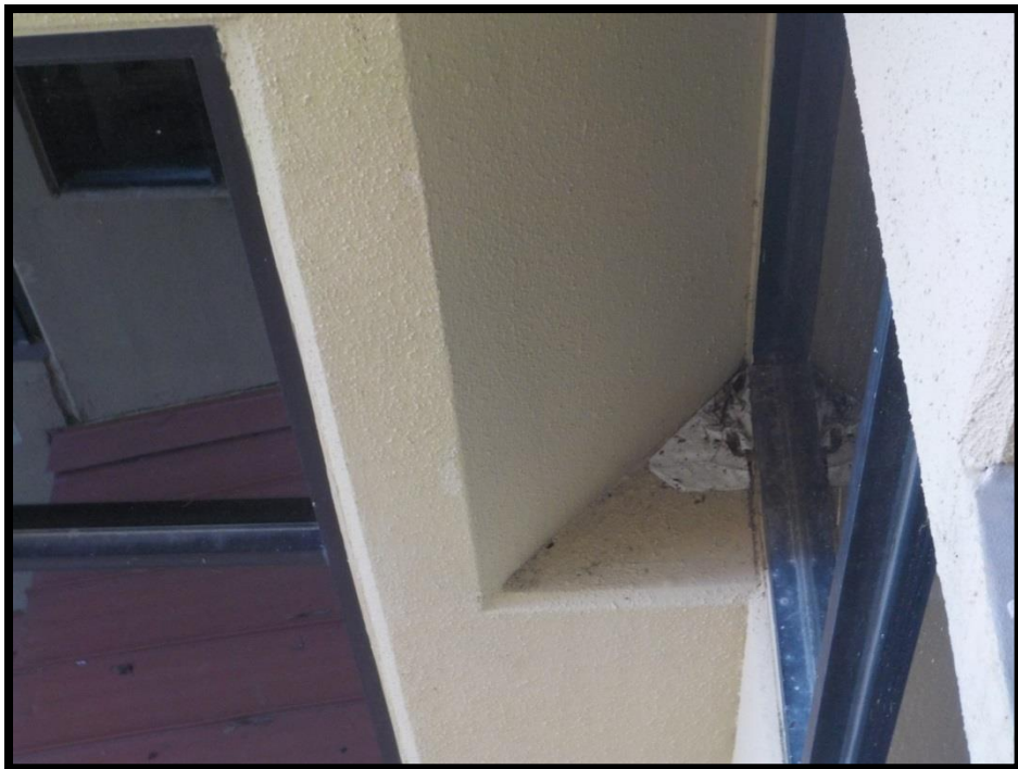
7 – Low slope edge that holds water at the elevator shaft.
