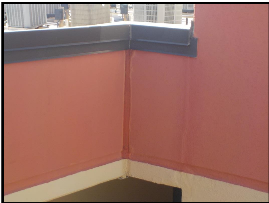
4 – Parapet expansion joint overview.
